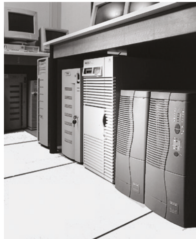
Fig. N32 UPS unit achieving dispoibility and quality of computer system power supply
