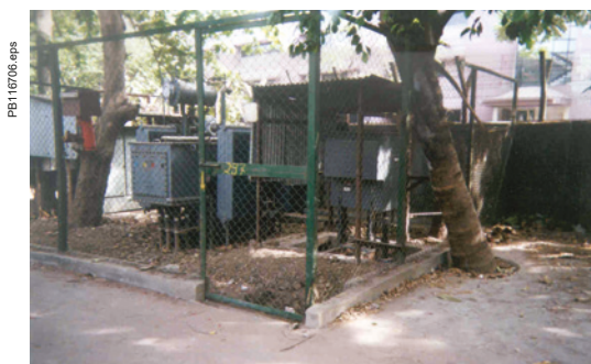
Fig. B53 Outdoor substation without enclosure
